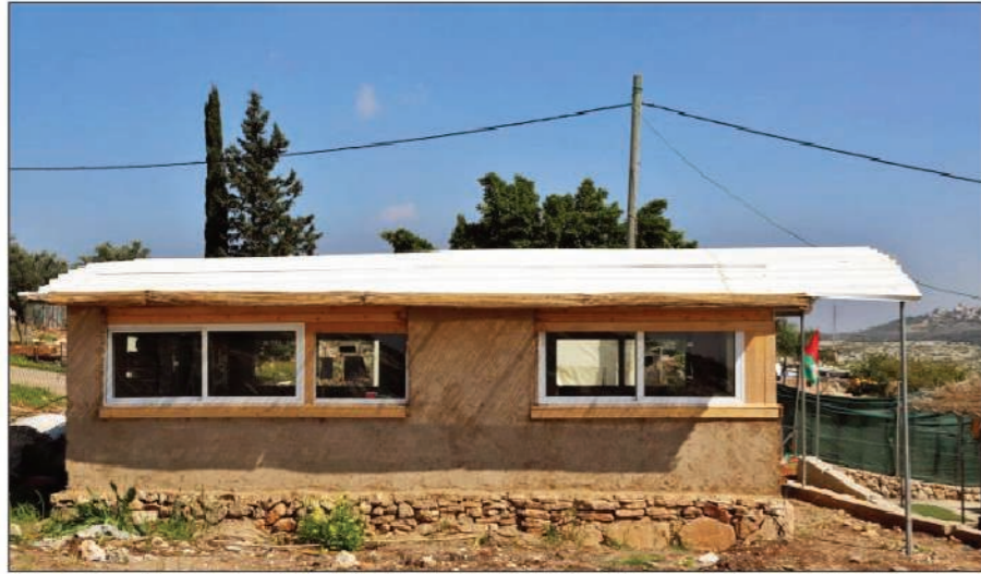
The school increases from 3 classes to 6 adding new services and teachers rooms, with no use of new land and reuse of materials in place.
