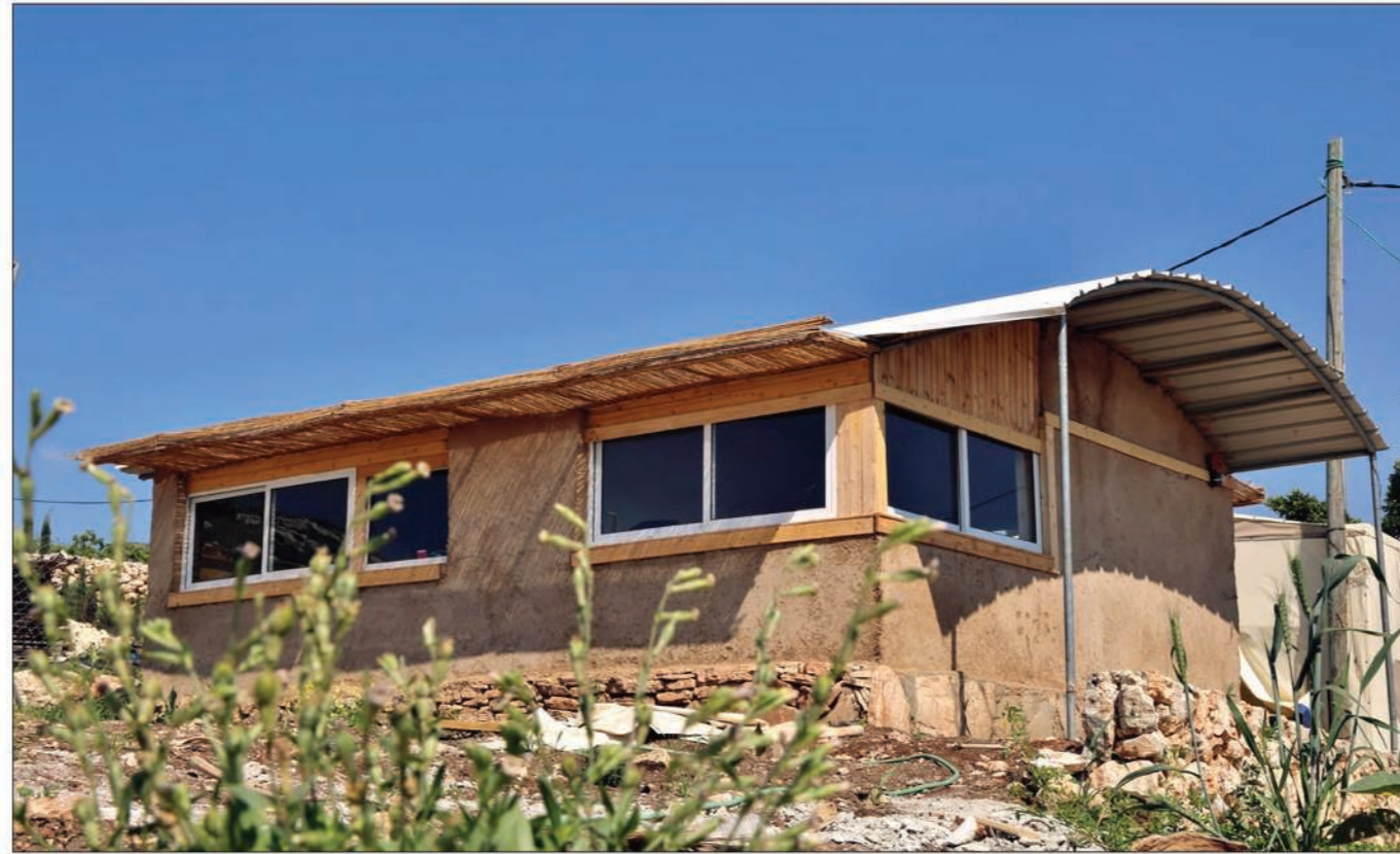
New permanent school with 6 classes, 2 teacher's room and toilet services. The specific strategy can become universal. It reuses and reinforces the original structure, transforming it in permanent spaces.
